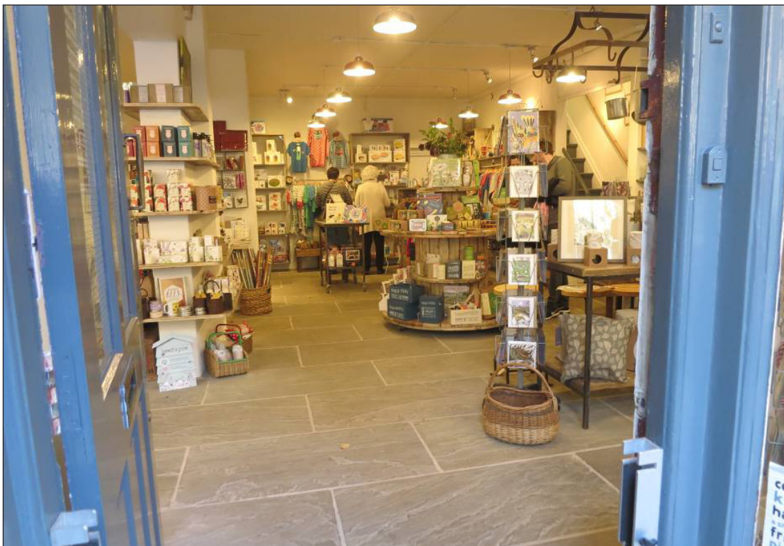
Figure 6: The timber floor was removed and replaced with stone flags.
