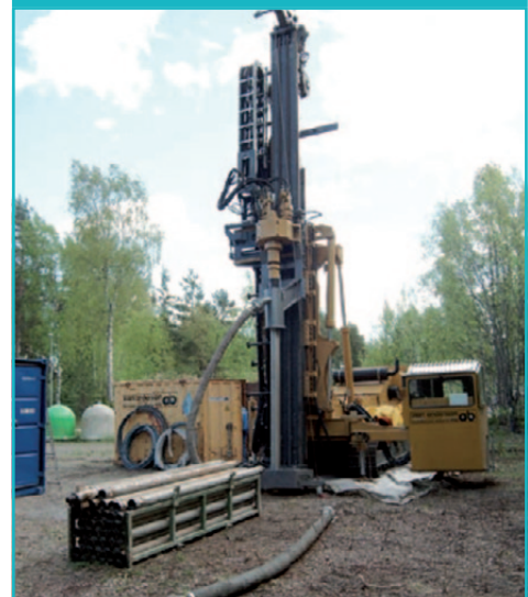
Figure 10.4: Borehole drilling in Sweden (source: SKB/Alf Sevastik Kustbild)
