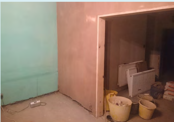
Re-plastering in the living room.
