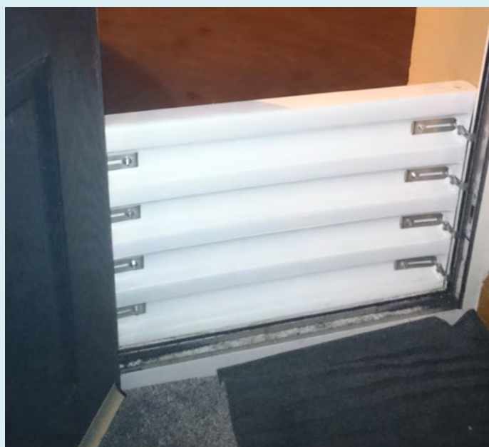
Above: flood doors fitted by previous owner
