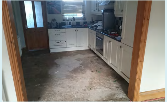
Tiles in the kitchen floor were stripped out and replaced.
