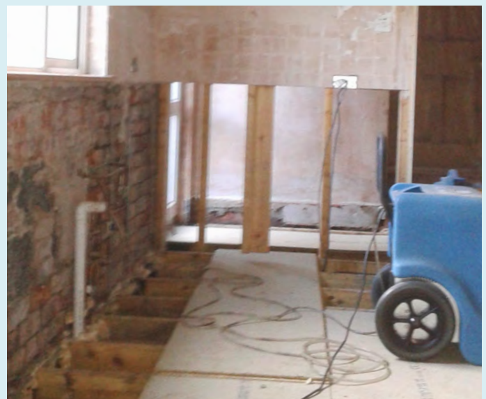
Drying out was by the gas central heating and dehumidifiers.
