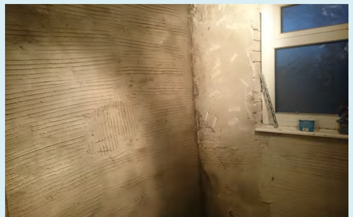
Bathroom tiles were also removed and replaced.
